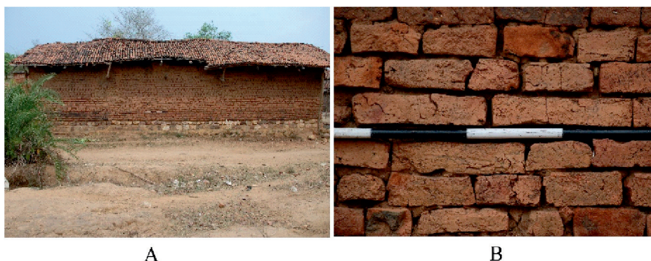
Fig. 9: Showing a tile-thatched house (A) the wall of which is constructed by using modern and Gupta period bricks (B)
